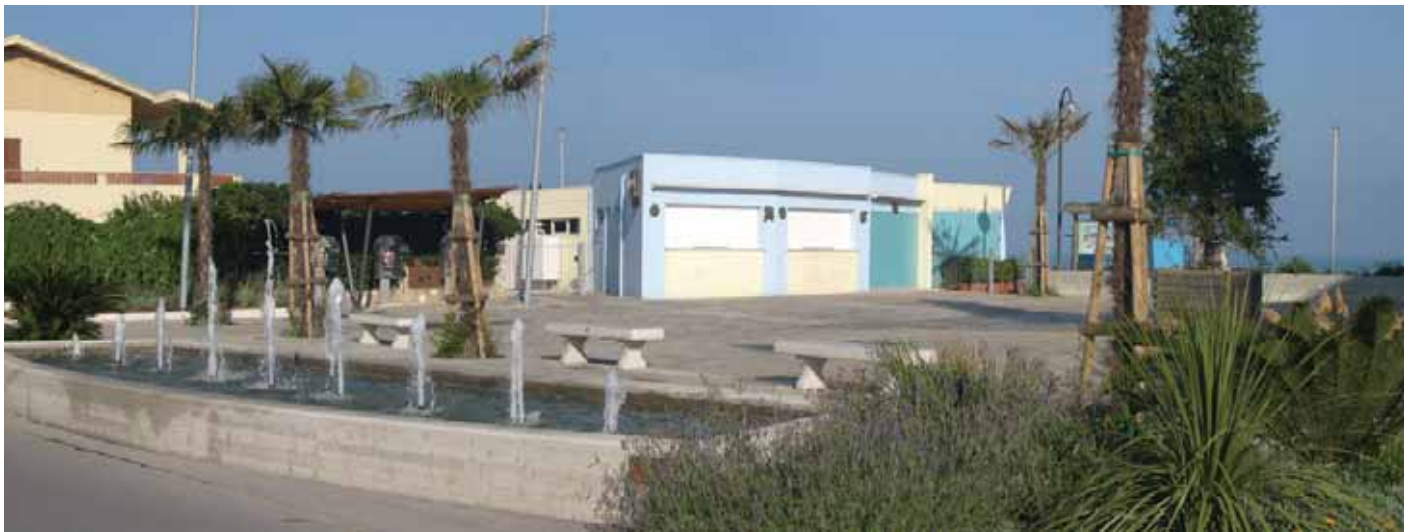
Photo 8 - The demonstrative project of Piazza Miramare on the seafront of Marcelli. The roofs of the telephone boots are made, as well as the ones of the other structures of the square, of photovoltaic modules.
